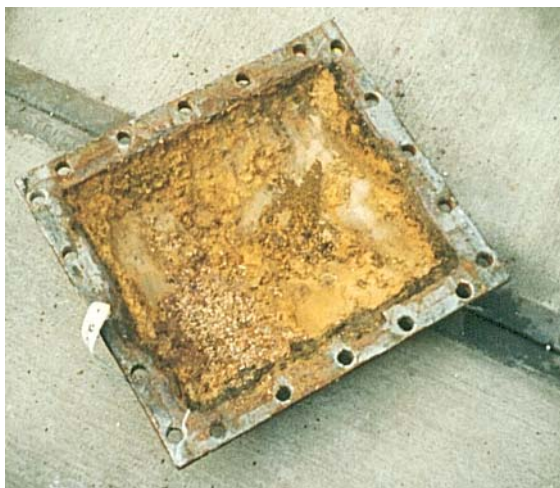
Photo 1: Cover of cooling system corrosion and scale deposit without Mexel ® 432 treatment
