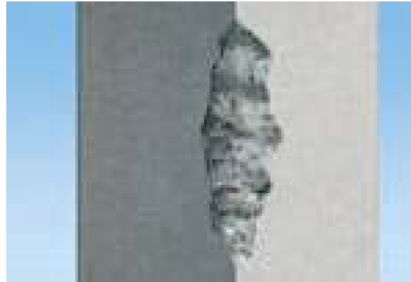
Difficult formworks removal
