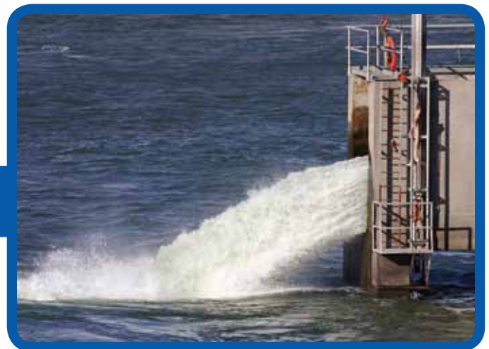
Power Station water outlet
