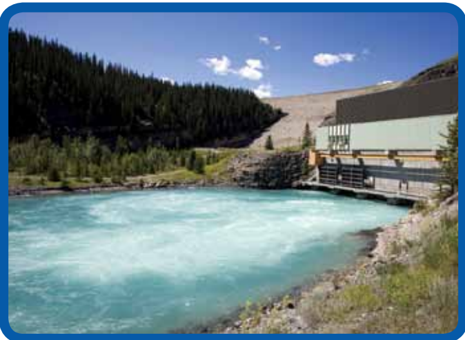
Power Station water outlet
