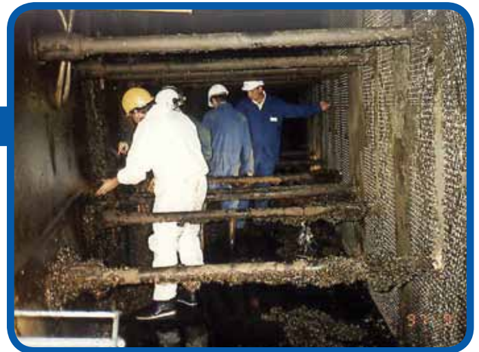
Power Station Flow 22 m 3 /s – Open cooling circuit, Sea Water - Treated with MEXEL
